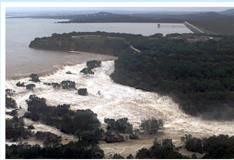
Canyon Reservoir spillway. During the flood of 1998, peak rainfall occurred downstream of Canyon Reservoir. In July of 2002, record rains filled the reservoir to capacity and the emergency spillway was used for the first time.
