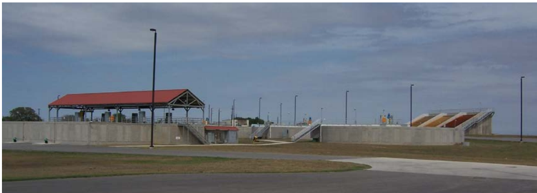
Figure 3: Water Treatment Plant (Morris, 2006)
